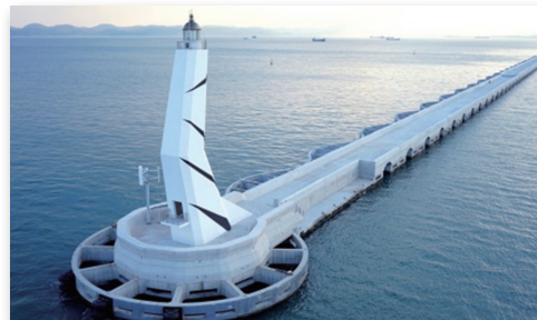
Pohang Yeongil bay breakwater
